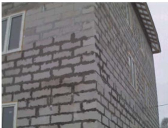
Figure 5. Heat-conducting fractions as brickwork joints.
