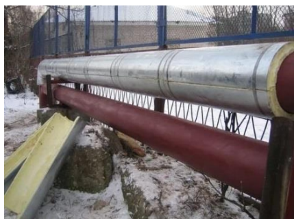
Figure 4. Image of a pipeline with a high-density polyurethane foam insulation.
