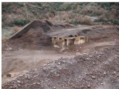
Figure 8. Halaköy Şubesi mercury mine loading dock with calcined tailings.
