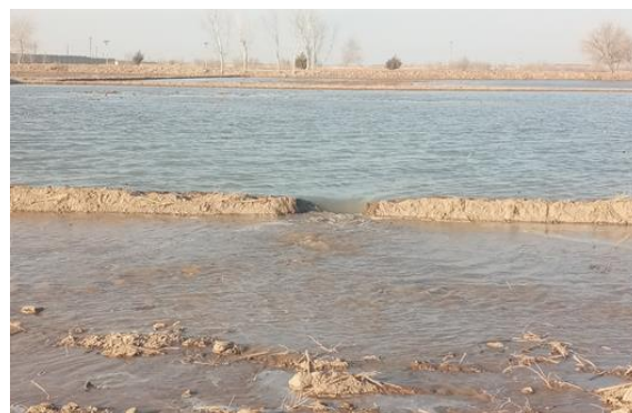
Figure 2. Water leakage to another part due to the rupture of the shell during the salting process.
