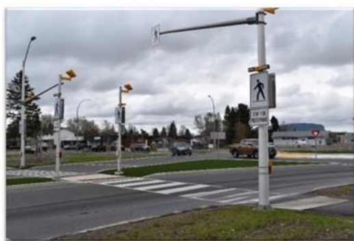
Figure 2. Rectangular Rapid Flashing Beacon (RRFB) with an Accessible Pedestrian Signal (APS) and push button on the pole, Thunder Bay.
