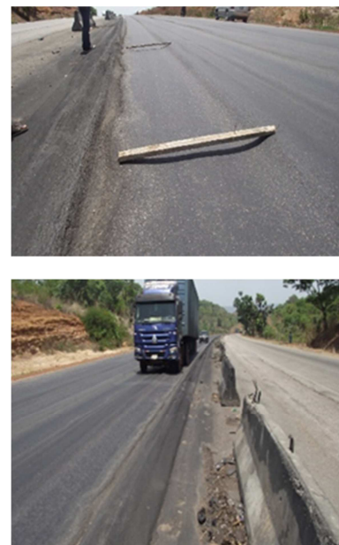
Figure 1. Pavement Damage on Lokoja-Abuja Expressway due to Overloading.
