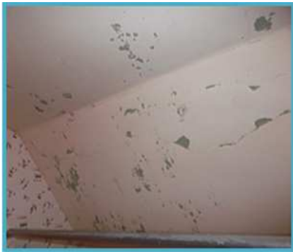
Figure 15. Crazing of Paint.
