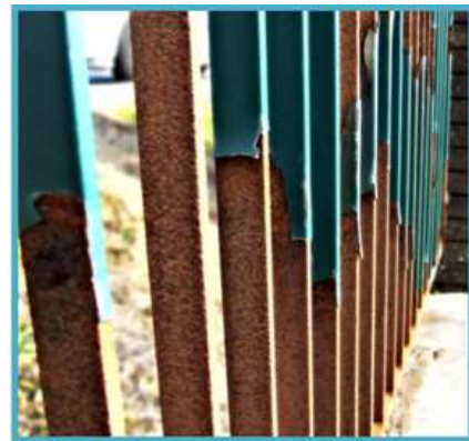
Figure 19. Flaking of Paint.
