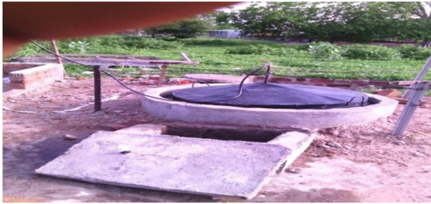
Figure 1. A 3m³ floating drum continuous biogas plant.
