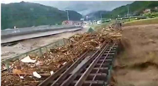
Figure 3. Wood debris accumulation on the railroad bridge.
