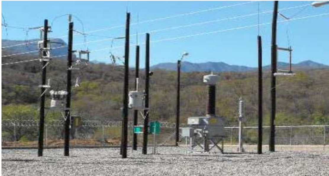
Figure 2. Auxiliary service voltage transformer (ASVT)
