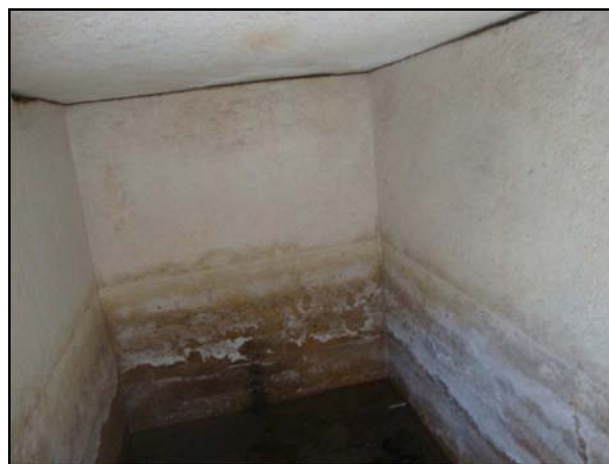
Figure 20. Shows growth of salts and algae inside the limestone's coffin.
