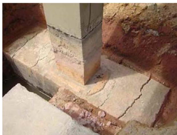
Figure 4. Fissure in block on two stakes, with dimensions 1 x 2,5m [25].
