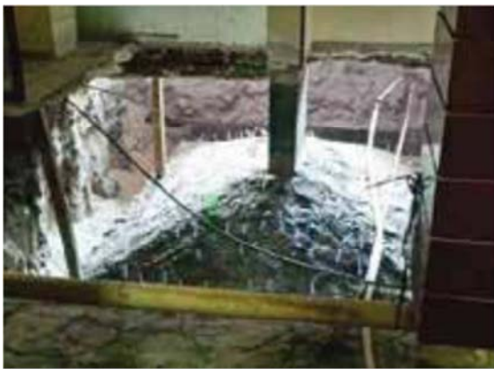
Figure 10. Low shoe bleeders [27].
