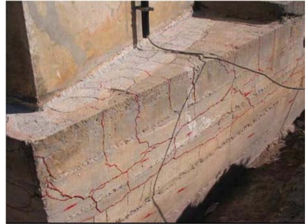
Figure 6. Upper and lateral block faces with cracks painted [25].
