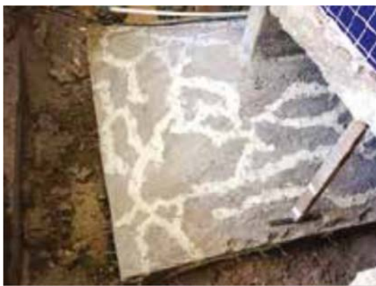
Figure 11. Cracks and fissures clogging [27].
