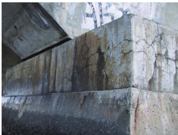
Figure 2. Signs of AAR in the central span support block of the Paulo Guerra Bridge [26].
