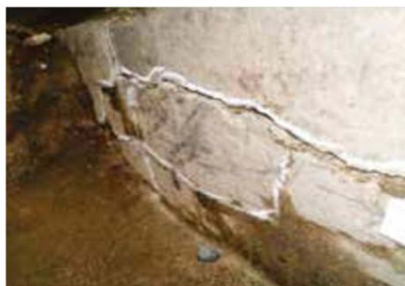
Figure 9. Low shoes with cracks in maps marked with chalk [27].
