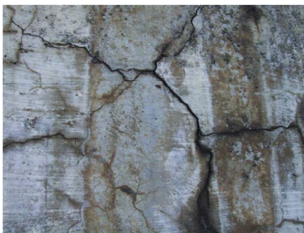
Figure 3. Crack in the shape of a map in the foundation block of the Paulo Guerra Bridge [26].
