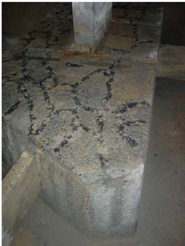
Figure 8. Foundation block with cracks already filled [25].
