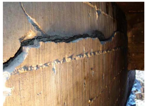
Figure 7. Horizontal crack with large opening and displacement [25].
