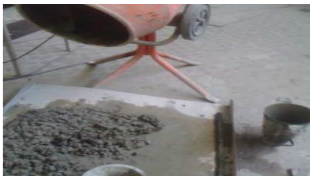
Figure 5. Mixing ingredients of concrete.
