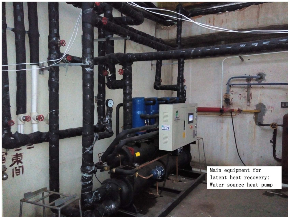
Figure 4. The main equipment for latent heat recovery in the test--water source heat pump.
