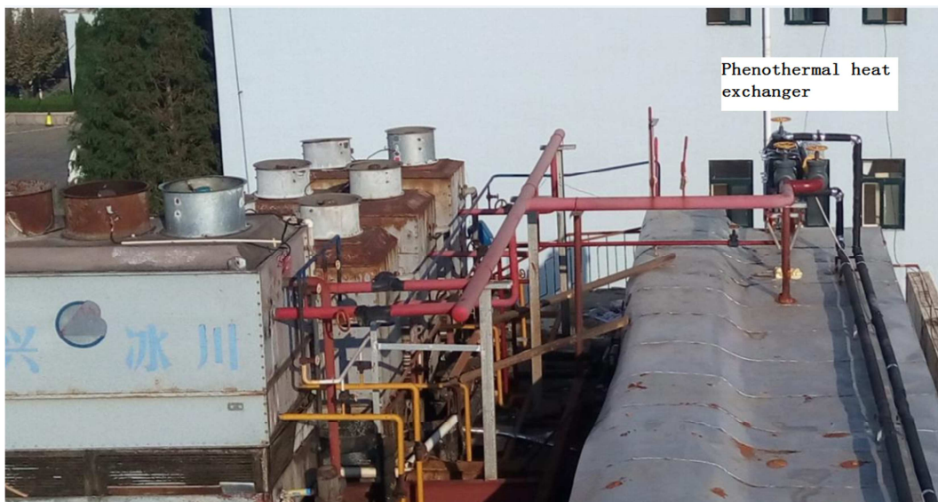
Figure 3. The main equipment for sensible heat recovery in the test - heat exchanger.
