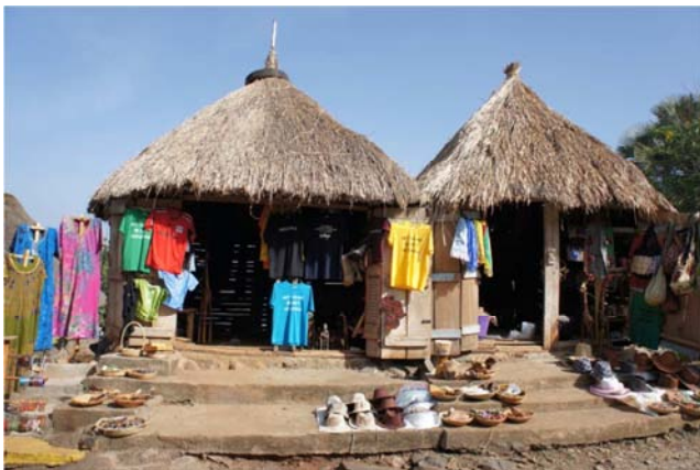
Figure 1. A commercial structure where many people could be taking shelter during a sudden thunderstorm. This is a typical sheltering structure for both housing and other use, in developing countries, which involve wooden or mudbrick walls with a combination of flammable thatch and wooden roof, often held down by stones. Components of the entire structure and its contents are inflammable.
