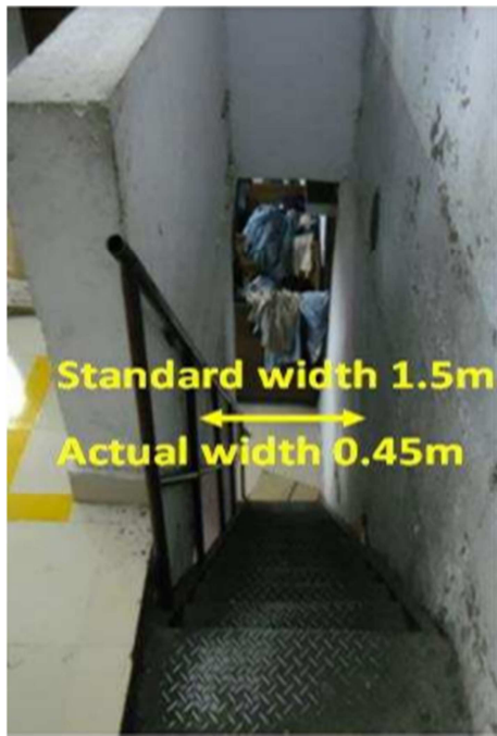
Figure 3. Hard factors: The stairway does not meet regulations [24].
