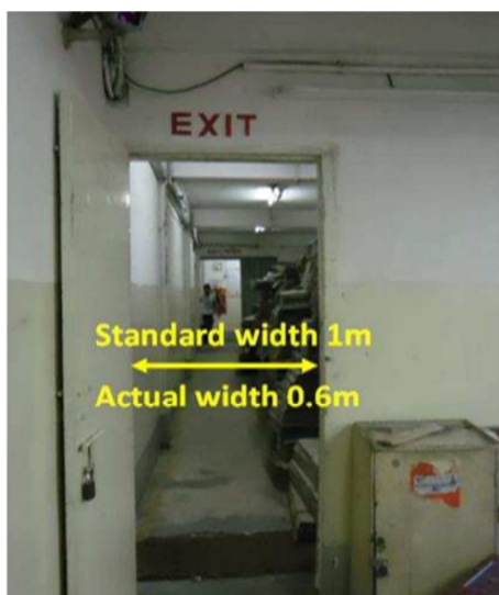
Figure 4. Hard factors: The entrance does not meet regulations [24].
