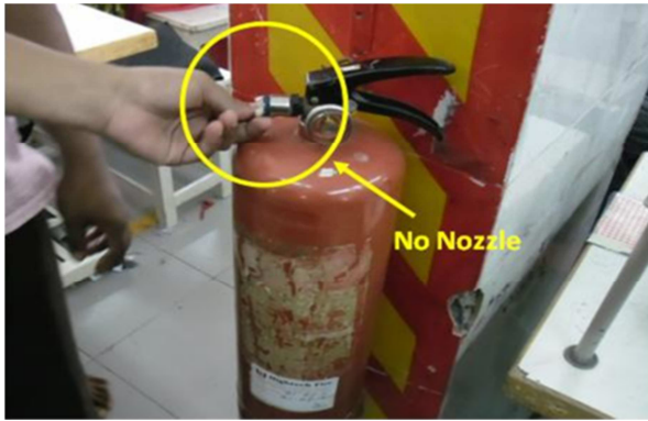
Figure 10. Soft factors: Fire extinguisher with no nozzle [23].
