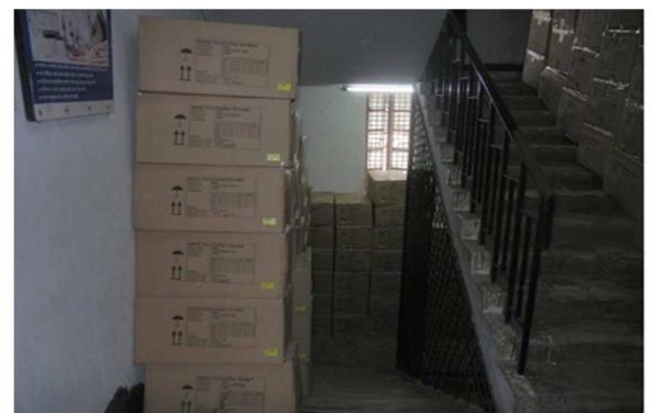
Figure 8. Soft factors: The stairway width meets regulation but is reduced in practice [24].
