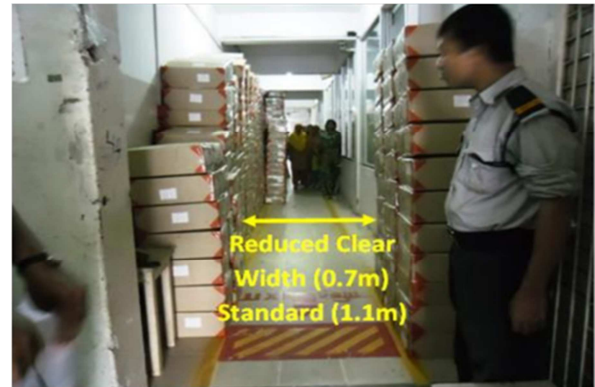
Figure 1. Soft factors: The clear width of an exit corridor reduced by piled-up boxes [23].
