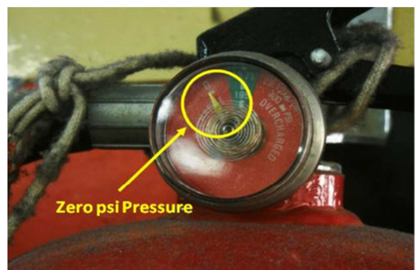
Figure 9. Soft factors: Fire extinguisher with zero operating pressure [23].
