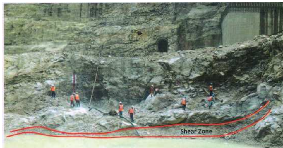
Figure 3. Shear Zone Right Side of Excavated Trench.
