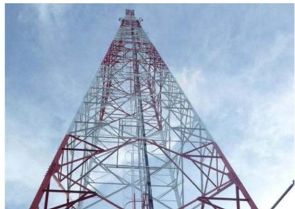
Figure 6. Square lattice tower with angle sections.
